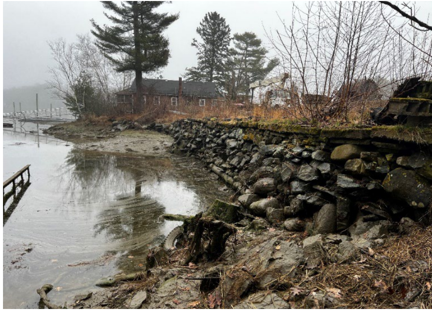
Photograph 5a: Looking south, view of cribbed stone retaining wall, from A-10 eastward (see Sheet 5); April 2024
